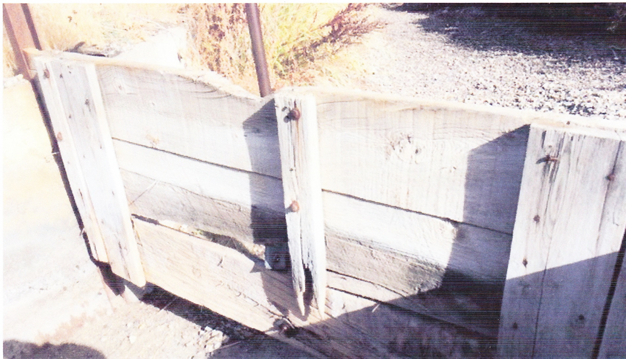
Take-out gate at the top of the Walker Lateral This wood may be 40 years old. Replacing it with steel.
