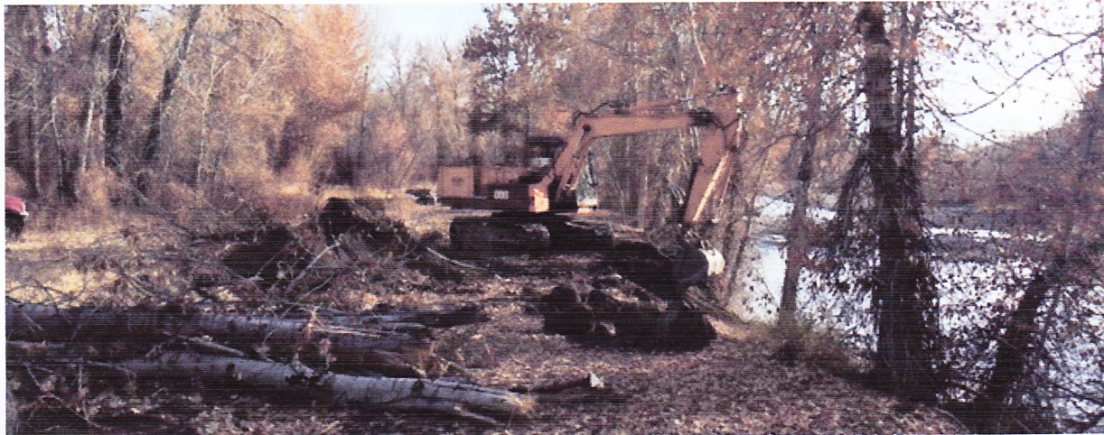
Keith breaking ground November 4
