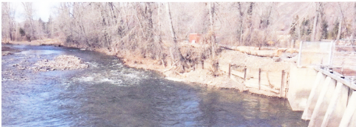
Replacing this dilapidated remnant from the past is underway
