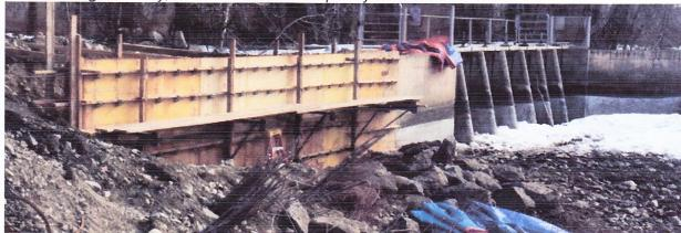
The New Mains Back to work, Mid March. An extension of the existing concrete wing-wall, on the upstream side, will provide further protection to the top of the Canal plus a transition from the new organic river bank into the old, very stable Main Headgate structure. The new
