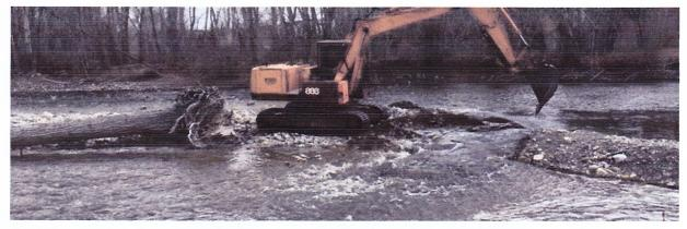
April 3 All ready for water! Keith opening up the coffer dam and allowing the river back over to our side.
