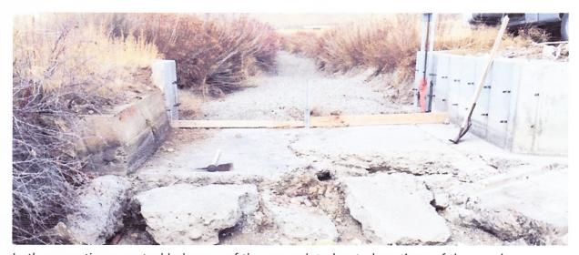
In the meantime: we tackled some of the more deteriorated portions of the canal infrastructure. The old floor, here is possibly around a hundred years old. In this case, there is a more recent wall on the left, and now a brand new wall on the right, put in by one of our water users along Kingsbury. Allowing these places to erode excessively would lead to unnecessary instability progressing up the canal bottom, and become increasingly difficult to repair.
