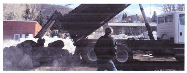
Rock hauled in It was placed deep under the bank and also up the slope to ensure stability of the embedded logs, roots, and willow bundles.
