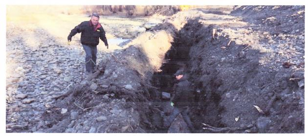
Embedding large rocks below the river bed to prevent any water from undermining the bank. The eastern bank of the river had been dried up by building a gravel bar up stream, to direct all flow towards the west side of the river.
