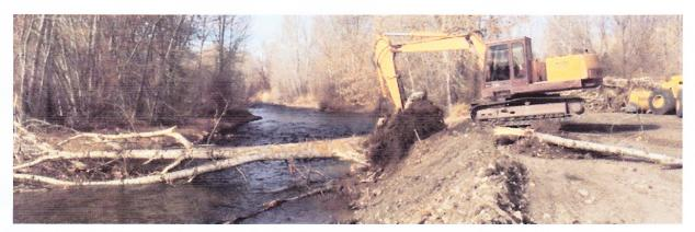
*Pulling with all his might.* Note the back end of the excavator off the ground as Keith pulled the last tree up the bank and out of the way. The roots of the trees, along with 20 foot lengths of the trunk attached, were buried back into the banks to provide very well anchored and solid interference for high velocity, highly erosive current.
