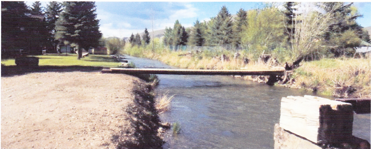
May 14 All done! New footbridge just above Ed's Drop
