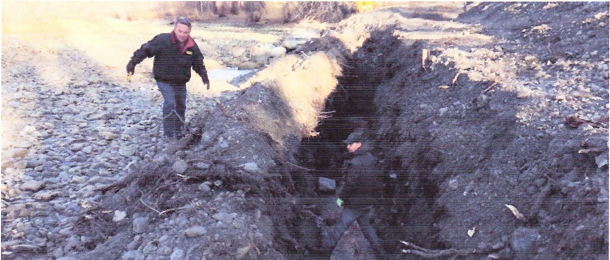
*Embedding large rocks below the river bed to prevent any water from undermining the bank. The eastern bank of the river had been dried up by building a gravel bar up stream, to direct all flow towards the west side of the river.*
