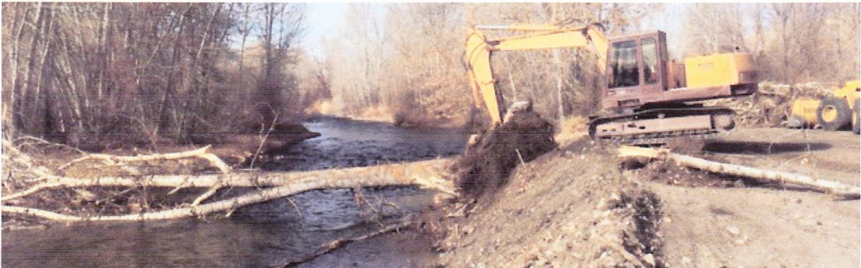
*Pulling with all his might.* Note the back end of the excavator off the ground as Keith pulled the last tree up the bank and out of the way. The roots of the trees, along with 20 foot lengths of the trunk attached, were buried back into the banks to provide very well anchored and solid interference for high velocity, highly erosive current.
