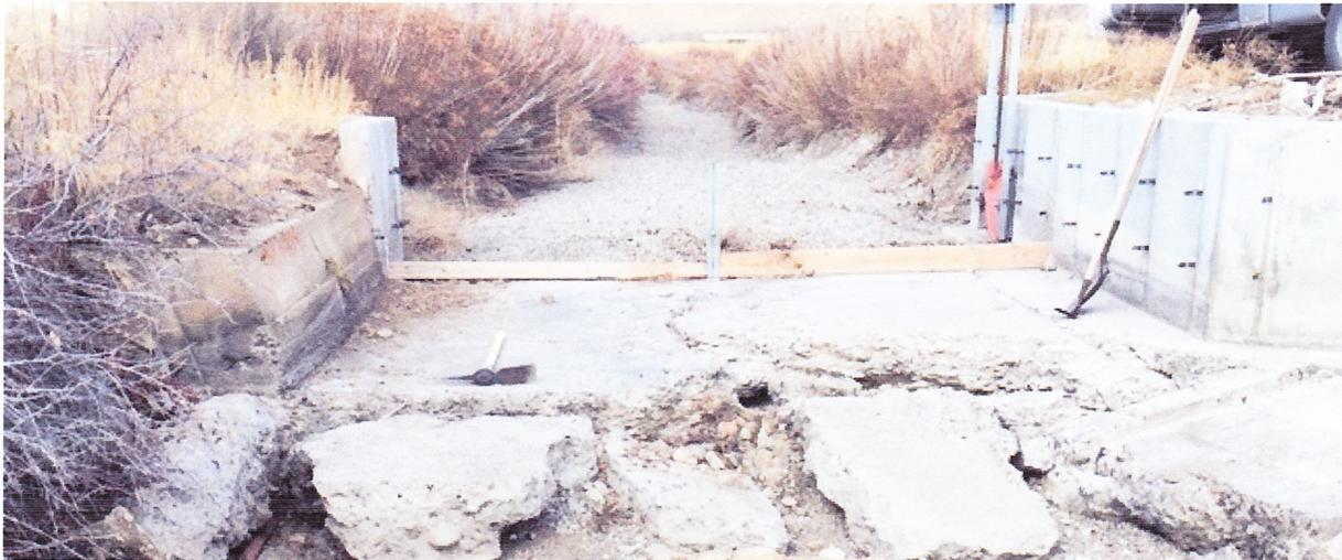
In the meantime: we tackled some of the more deteriorated portions of the canal infrastructure. The old floor, here is possibly around a hundred years old. In this case, there is a more recent wall on the left, and now a brand new wall on the right, put in by one of our water users along Kingsbury. Allowing these places to erode excessively would lead to unnecessary instability progressing up the canal bottom, and become increasingly difficult to repair.
