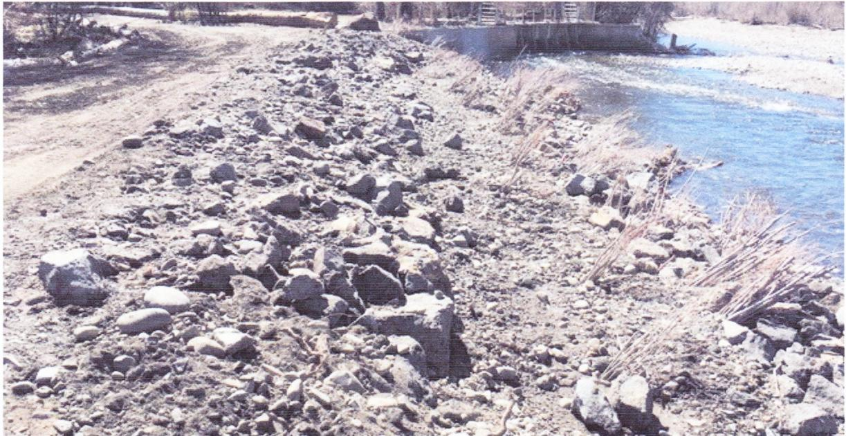
...*nice finishing touch*... he then took the last two loader-bucket loads of remaining rocks, sand, and gravel, and casually sprinkled it, haphazardly, over the bank, filling all the little gaps and cracks and giving the whole thing a slightly less manicured look while anchoring it all in place. I like it! Now all we need is a little high water to test it out. Not too likely, this year, I'm afraid..
