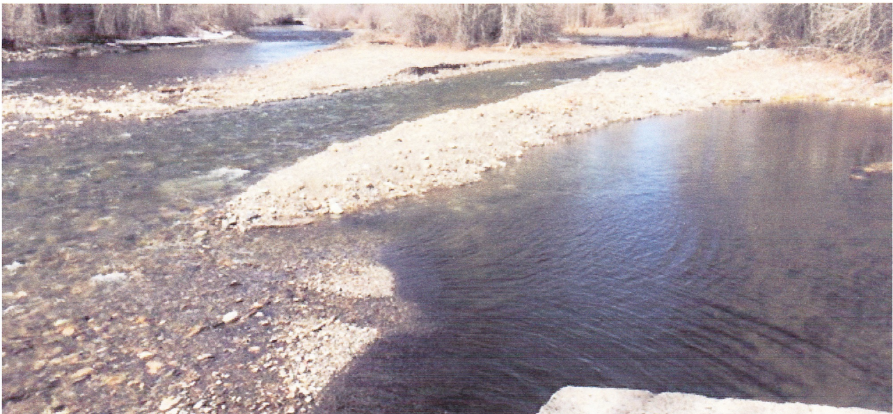
The remnant of our "in-river" coffer dam, built last Fall to dry out our Main Headgate. It served us well, and was only breached after two inches of rain fell last week.
